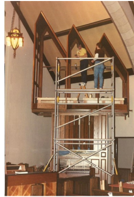
Building the framework for the organ pipes.
